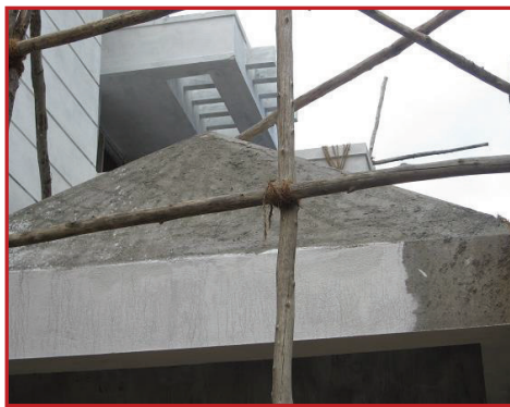
SLOPED ROOFS WATERPROOFING
